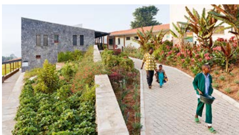
The 40-bed Butaro Hospital in Butaro, Rwanda.
