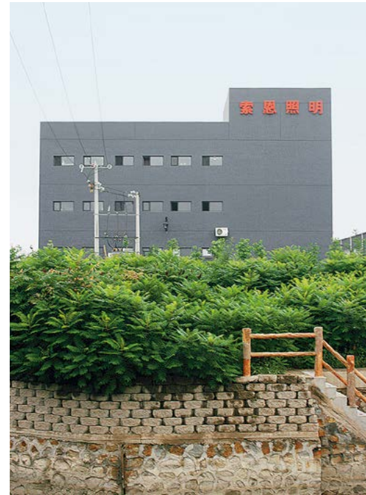
External view of the new plant in Tianjin.
